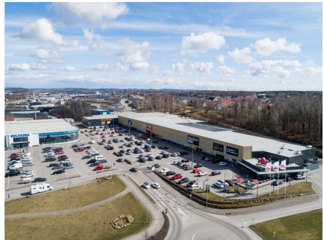
Retail property, Varberg, Sweden.
