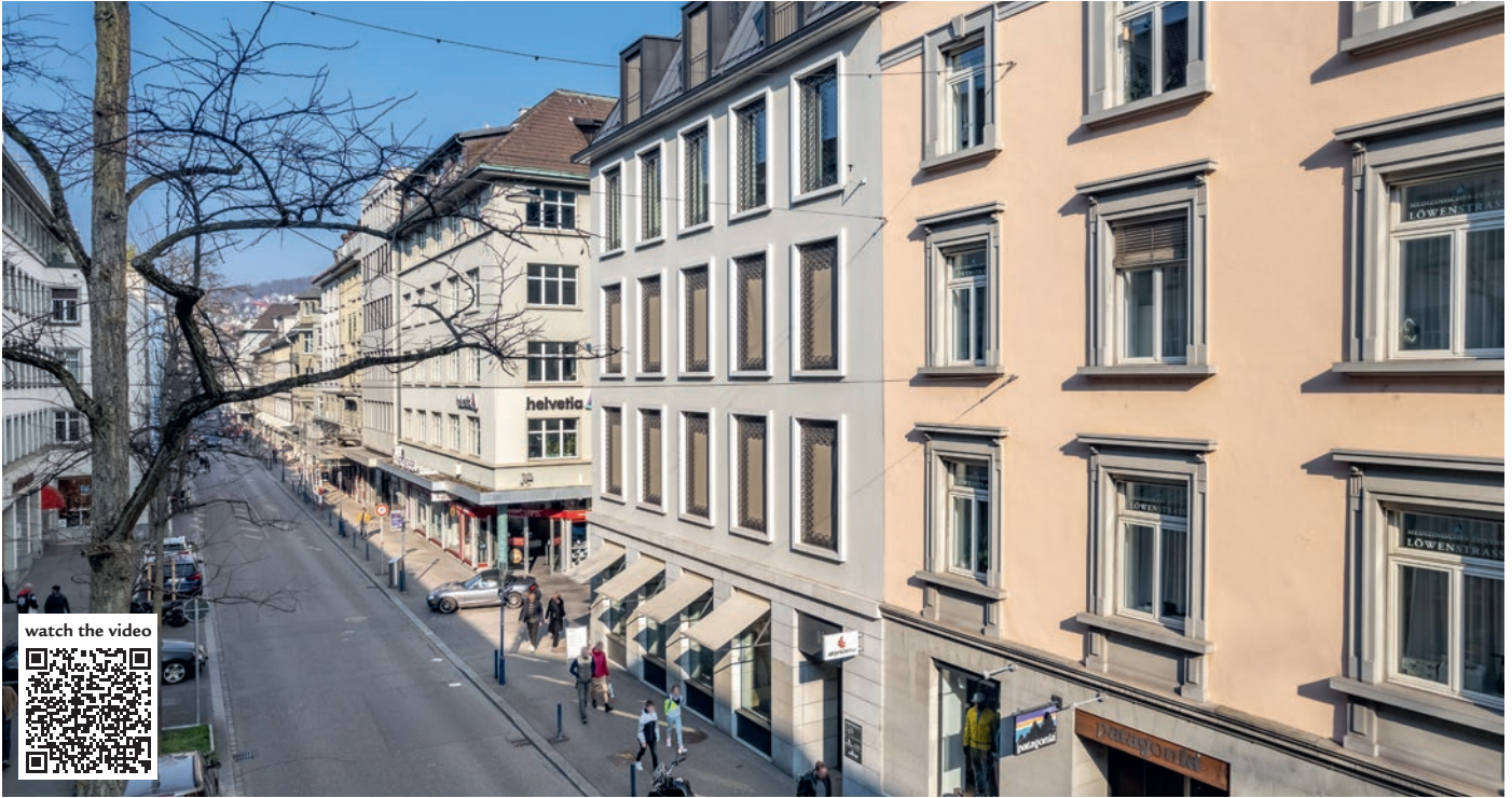
Löwenstrasse is a popular shopping street in the heart of Zurich with a wide range of stores. Source: Fotowerder
