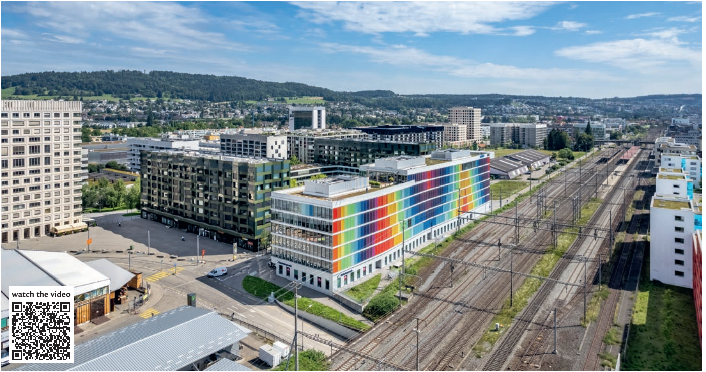
The roof is accessible and houses a terrace for tenants. Source: Fotowerder
