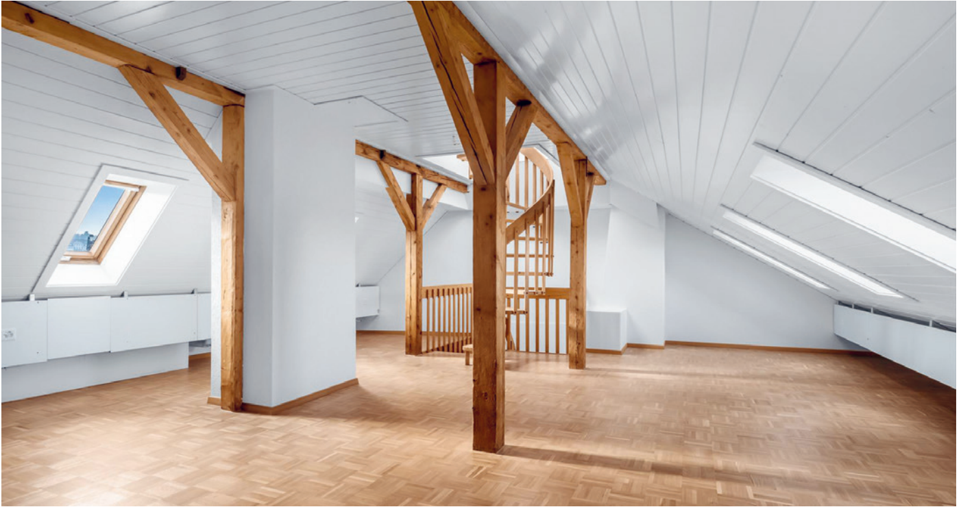
A room with a view: carefully refurbished, with a view over the border. Source: Fotowerder
